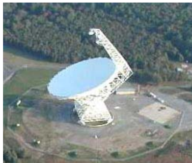
The Robert C. Byrd Green Bank Telescope (GBT), the world's largest fully steerable radio telescope, has 2004 individually adjustable panels. These reflective panels are mounted at their corners on actuators (drive pistons), which can make tiny adjustments to the positions of the panels, keeping the telescope perfectly in focus. Photograph courtesy NRAO.
