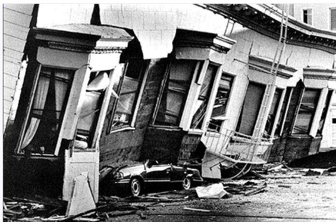
An apartment building in San Francisco's Marina District was thrown from its foundation and crushed a car in the 1989 magnitude 7.1 earthquake. The Marina District was the scene of voracious fires caused by broken gas lines. Photo by Vince Maggiora.
