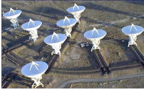
Small section of Very Large Array (VLA) radio telescopes, which move on tracks in coordination together in Datil, New Mexico. Image courtesy VLA.
