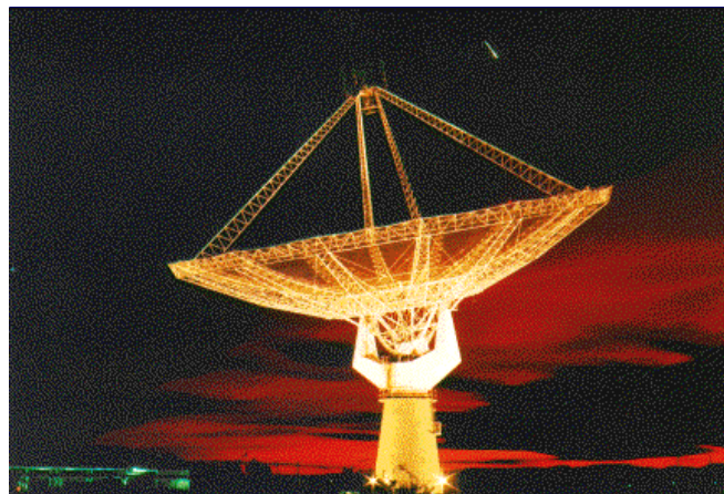
Giant Metrewave Radio Telescope (GMRT), near Pune in Maharashtra, India. GMRT is the world's largest radio telescope at meter wavelengths. It consists of thirty antennas of 45 meter-diameter spread over a 25 kilometer region and operating at wavelengths of 20cm, 49cm, 90cm, 128cm and 200cm. Image courtesy GMRT.
