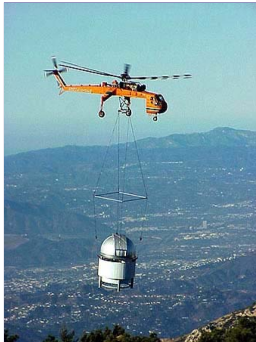
Skycrane hauling up interferometer housing at Mt. Wilson Observatory in Los Angeles, California, in 1998. Image source: Erickson Air-Crane, Inc.
