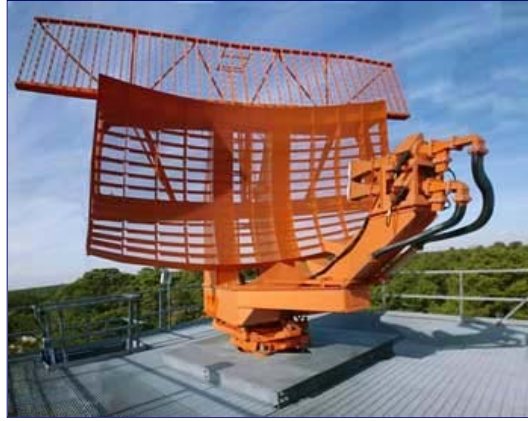
This ASR-9 radar antenna system is a typical ground radar installed at air traffic control facilities. The ladder-like top section is the secondary surveillance radars (SSR) directional antenna, which interrogates and listens for any replies. The remainder of the assembly makes up the primary surveillance radar (PSR) antenna. The system consists of transponders, which are automatic devices that receive an interrogation, decode it, decide whether to reply, and then respond with the requested information when appropriate. Image source FAA .
