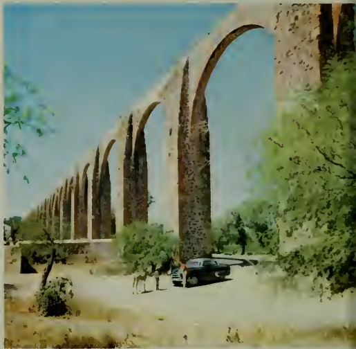
The aqueduct of Queretaro in Mexico was built in the early 1700's by the Spanish colonists. Its terra cotta pipes are still used today, suggesting what a high degree of development the vigorous Spanish colonization reached.
