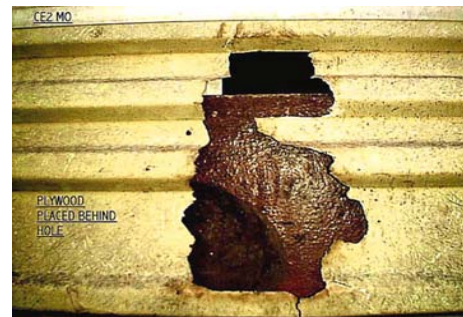
Closeup of door damage. Plywood has been placed behind the hole.
