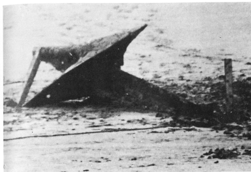
V Allan Beckett's kite anchor used to moor floating roadway
