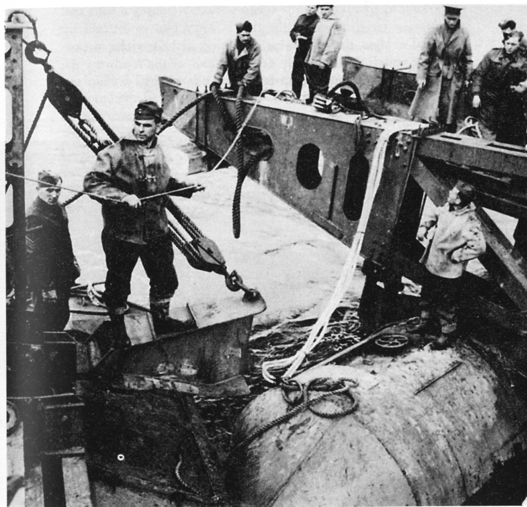
III Linking spans of the floating roadway, using erection tank (Public Record Office)
