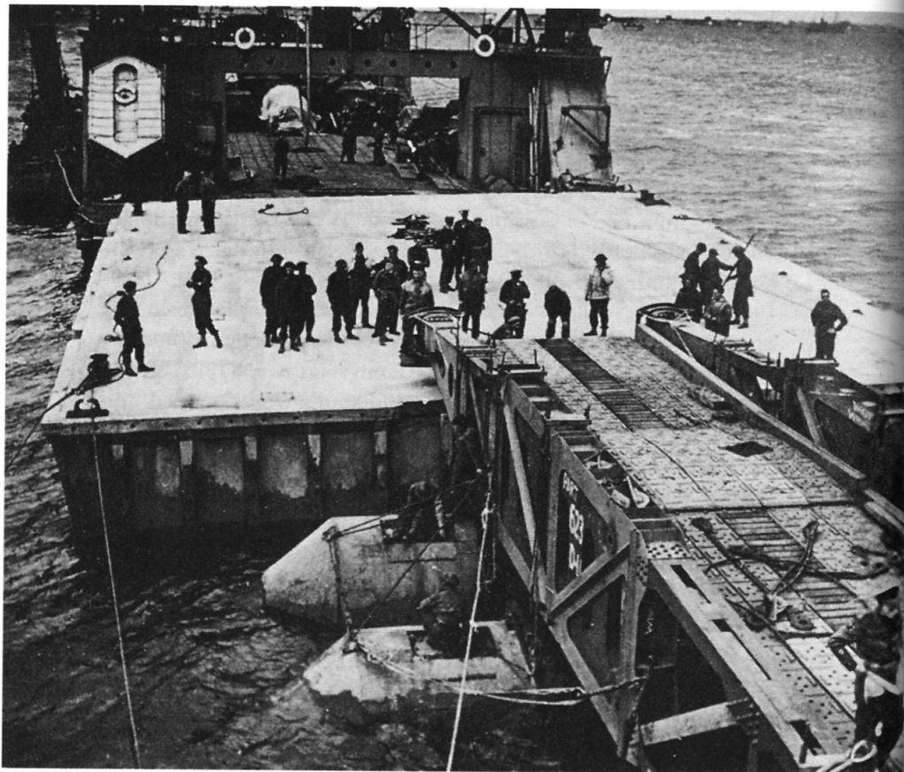
VIII Intermediate pontoon linked to spud pontoon to form enlarged pierhead
