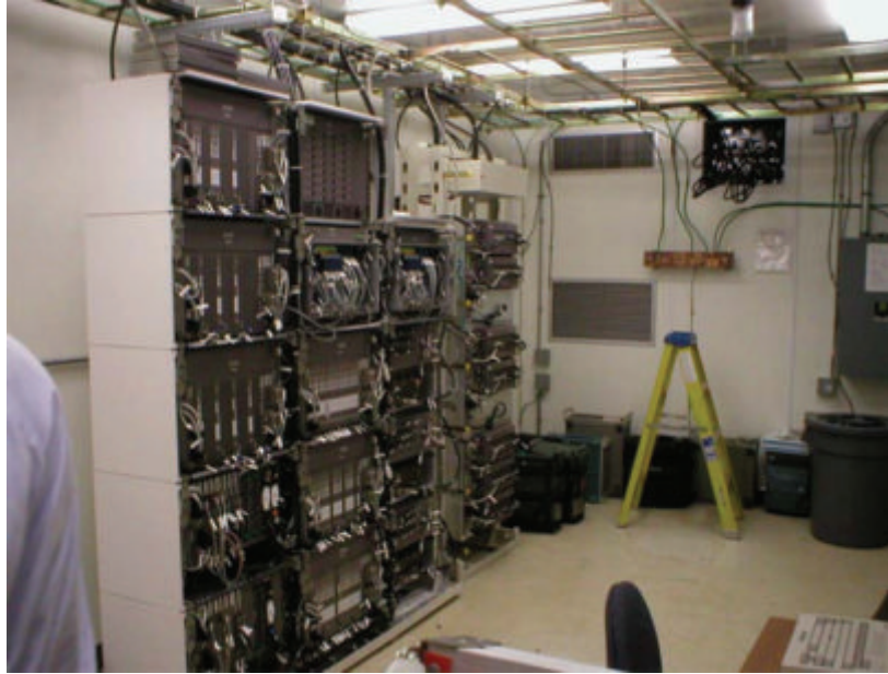
Figure 3-4. Cellular Base Station Equipment
