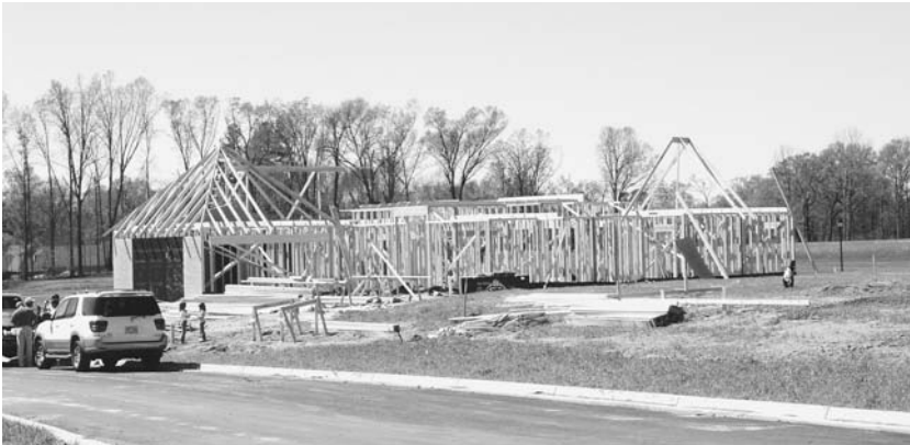
At the early stages of construction, this house's “skeleton” is a frame made of wood. (Kyle Kirkland)
