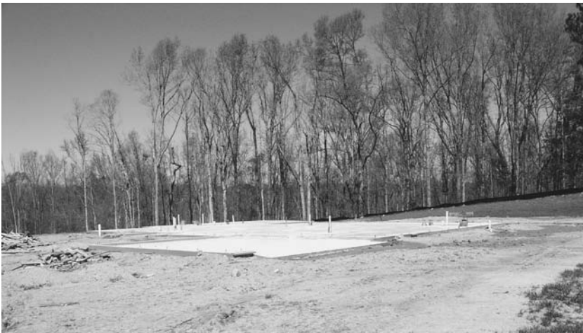
Concrete is often used for a building's foundation. A house will be built on top of these concrete slabs. (Kyle Kirkland)
