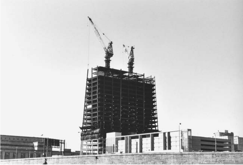
A steel frame for a skyscraper goes up in Philadelphia, Pennsylvania. This building will become the Cira Centre, as shown in the next figure. (Kyle Kirkland)
