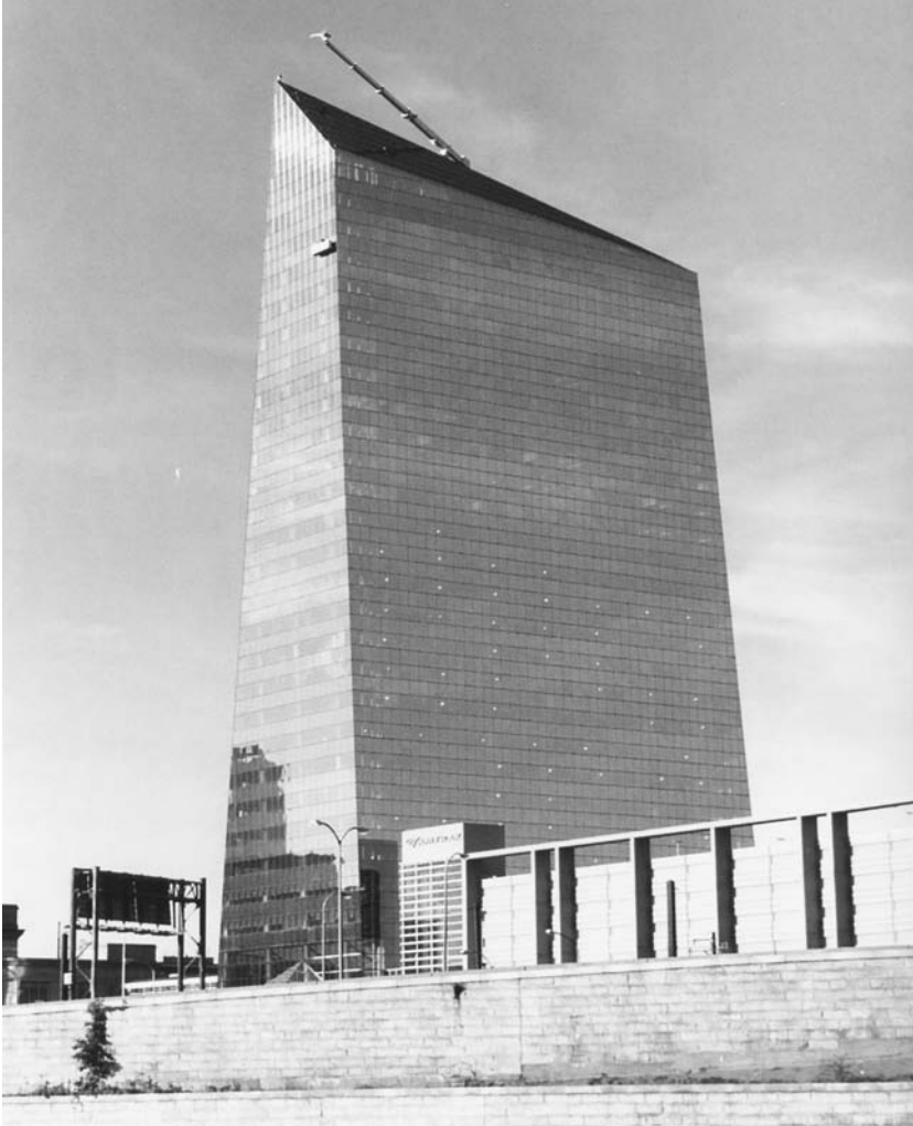
The nearly finished Ciria Centre is 436 feet (133 m) tall. The glass and plastic sides need not bear much weight, since the steel frame of the structure provides most of the support (see the previous figure). ( Kyle Kirkland )
