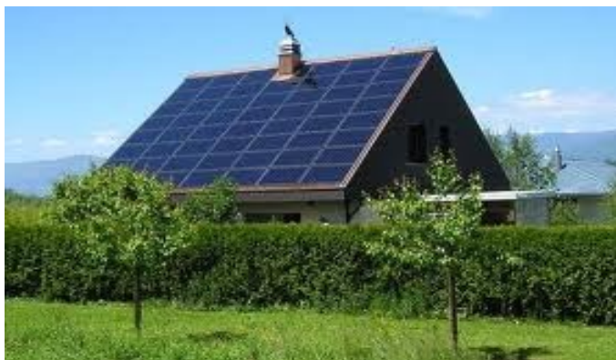
Illustration 16: Solar Roof Panels
