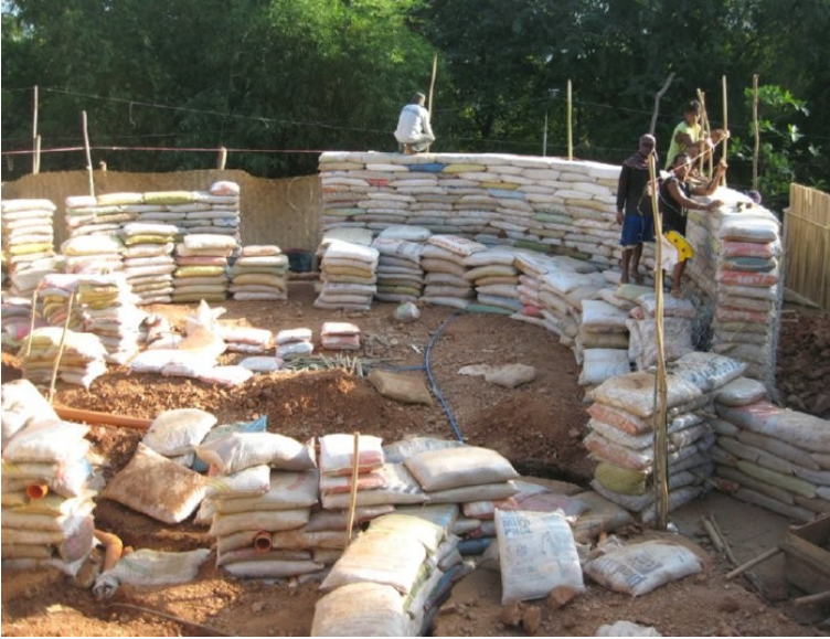
Illustration 8: Sandbag Construction
